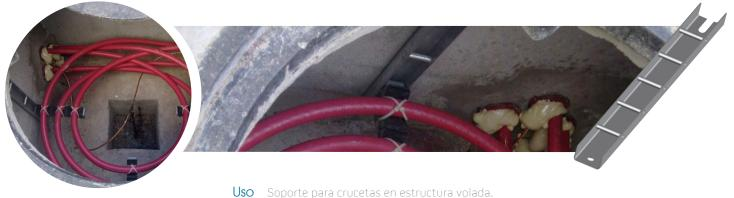
Mat T1: Angulo L1 50.8 mm x 4.76 mm. Solera 38.1 mm x 6.3 mm. T2: Angulo L1 38.1 mm x 4.76 mm. Solera 38.1 mm x 63 mm.
